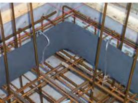
CEMflex can easily be bent on side up to 90 degrees and more!
