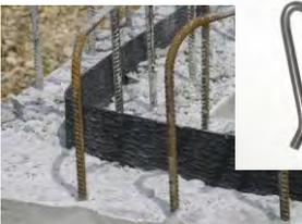
CEMflex VB can also be stuck into the fresh concrete. The overlappings have to be fixed only by using the CEMflex clip. The overlapping has to be at least 5 cm; gluing the overlappings is not required!
