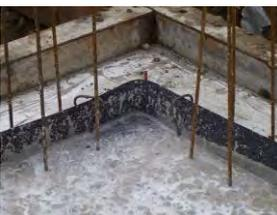
CEMflex VB properly embedded in the fresh concrete / first concrete section (a minimum of 3 cm concrete cover is required).
