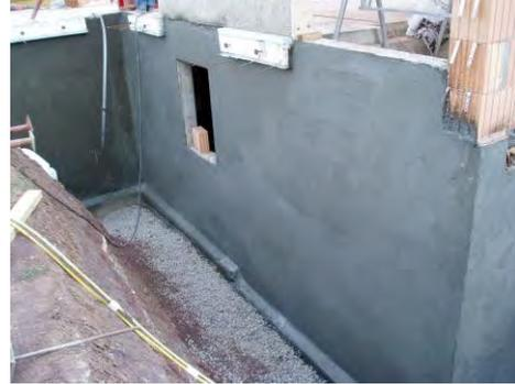
**Amount required:** Approx. 3 kg/m<sup>2</sup> against ground dampness and non-pressure water flow. Approx. 4 kg/m<sup>2</sup> against pressure water flow. The amounts given refer to the dry mortar.
